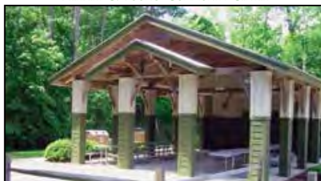
BOND PARK SHELTER
