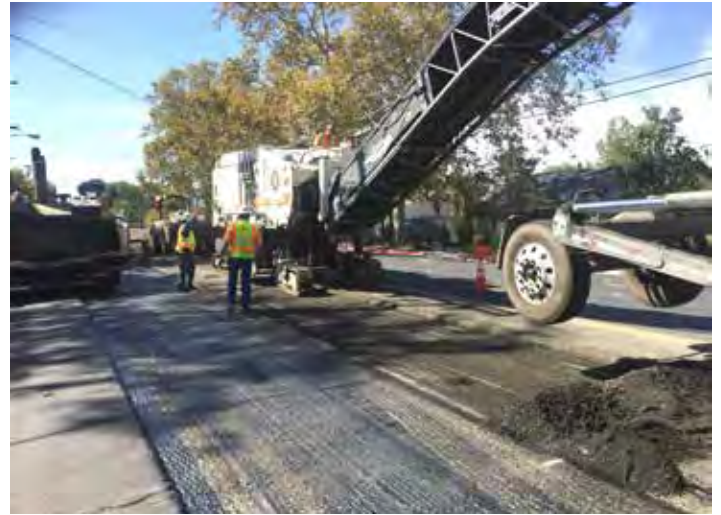
A crew works on one of the many streets improved last year as part of the Measure Q Pavement Repair Project
