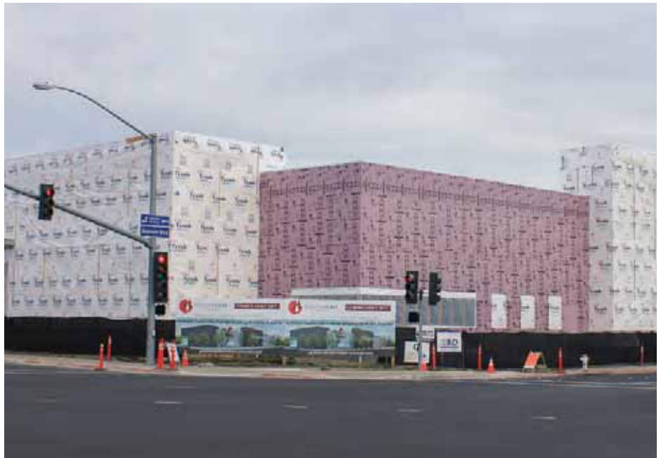
Golden State Lumber is under construction at Diamond Boulevard and Burnett Avenue
